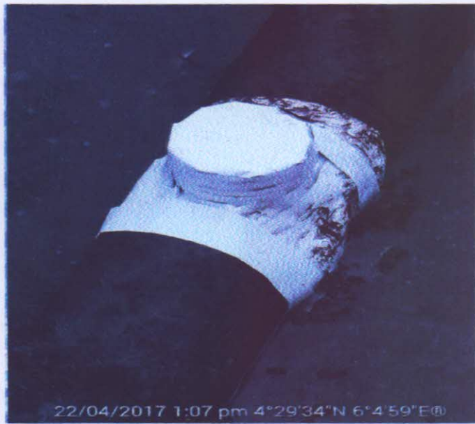
Figure 2: Coned after repair on the pipeline.
